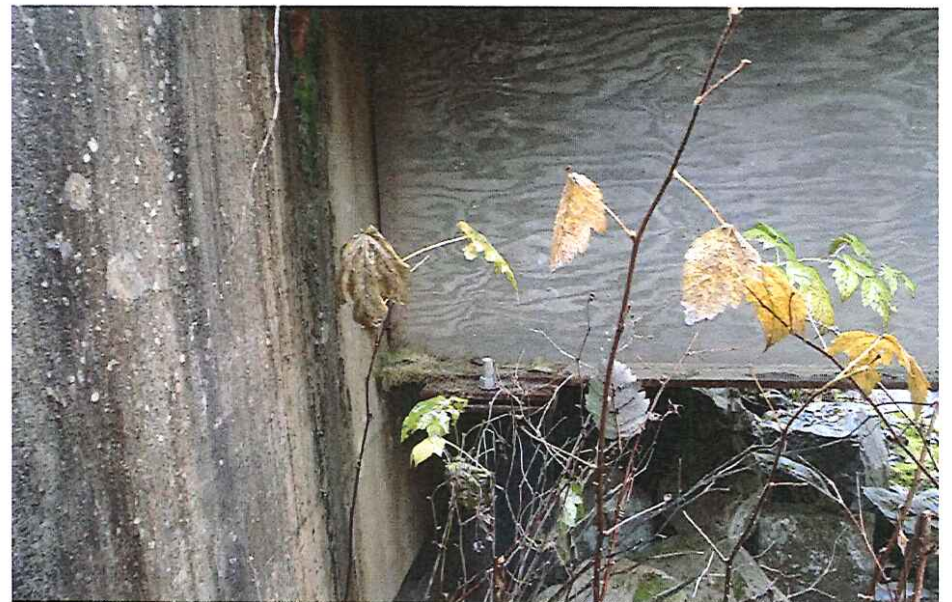
CK2067 Left Abutment bearing
