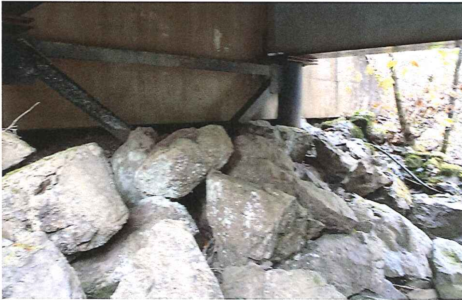
CK2067 Left Abutment
