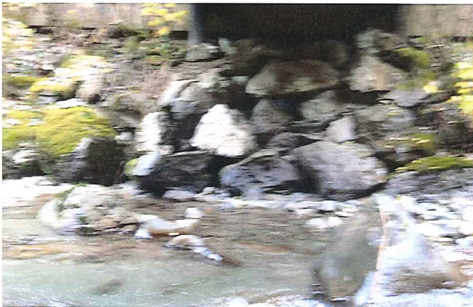
CK2067 Right Abutment
