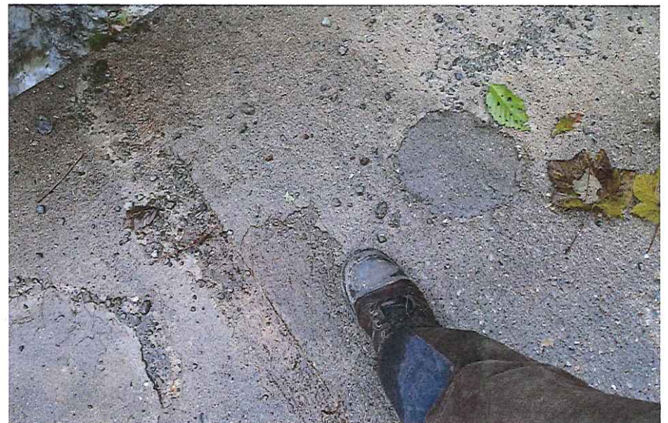
CK2067 Grout Pockets and joints
